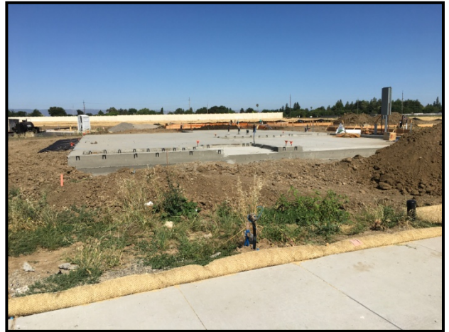
Home construction underway
