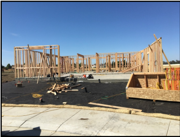
Home construction underway
