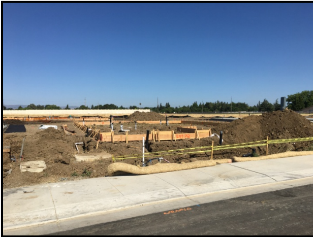
Home construction underway
