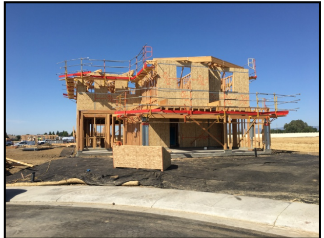
Home construction underway
