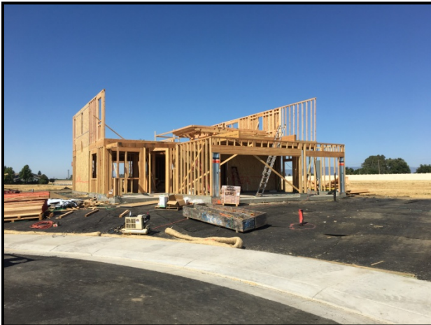
Home construction underway
